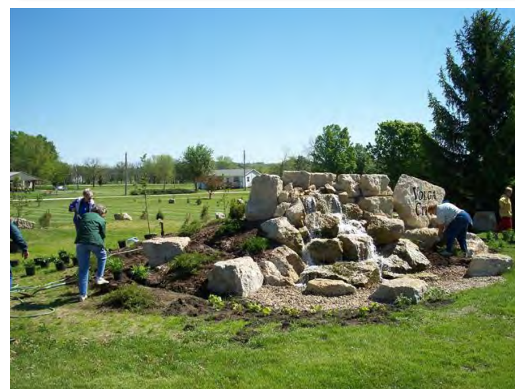
Volunteers constructing the sign
