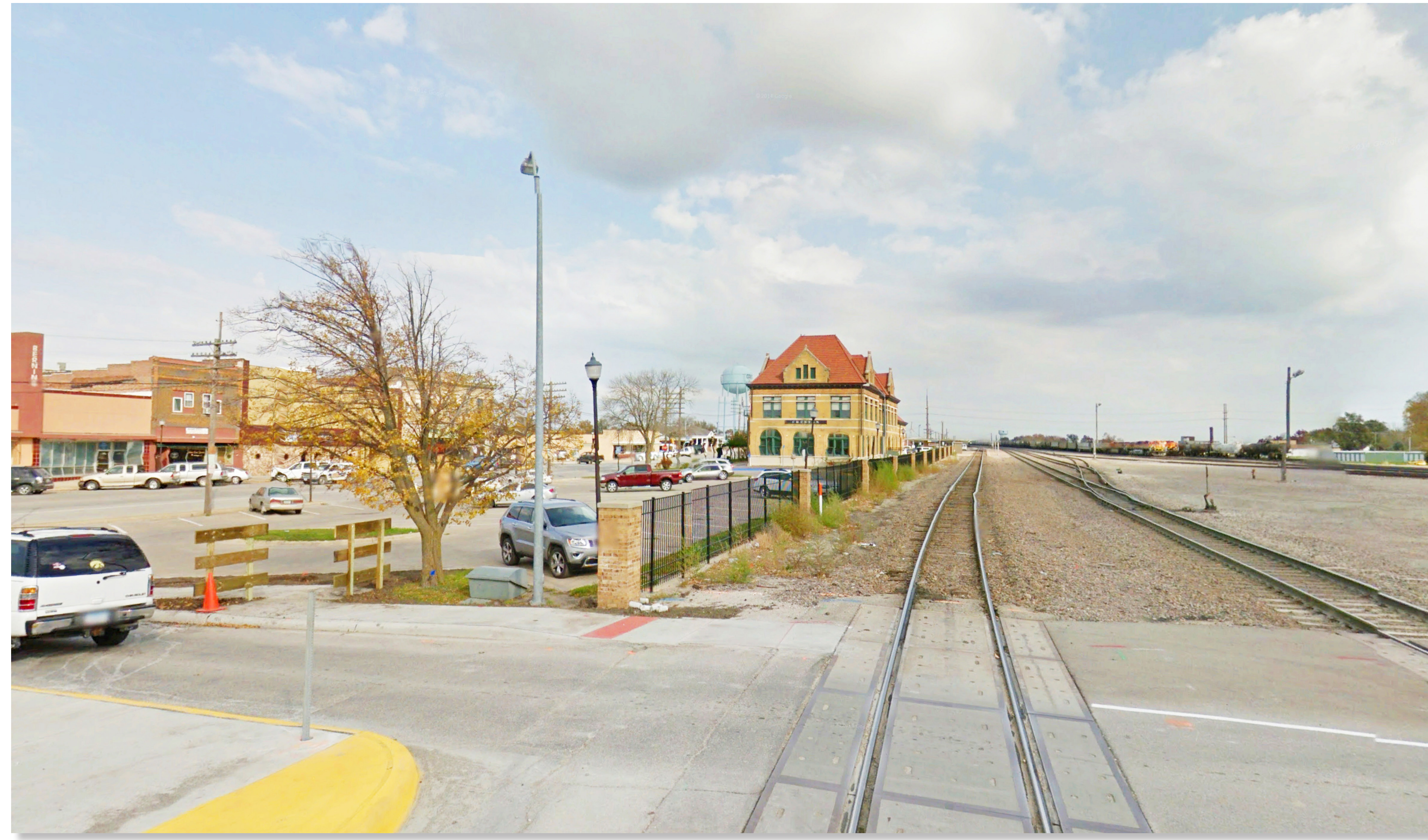
Railway corridor near city hall after project completion in 2006
