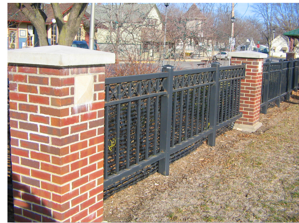
Completed fencing and brick pillars
