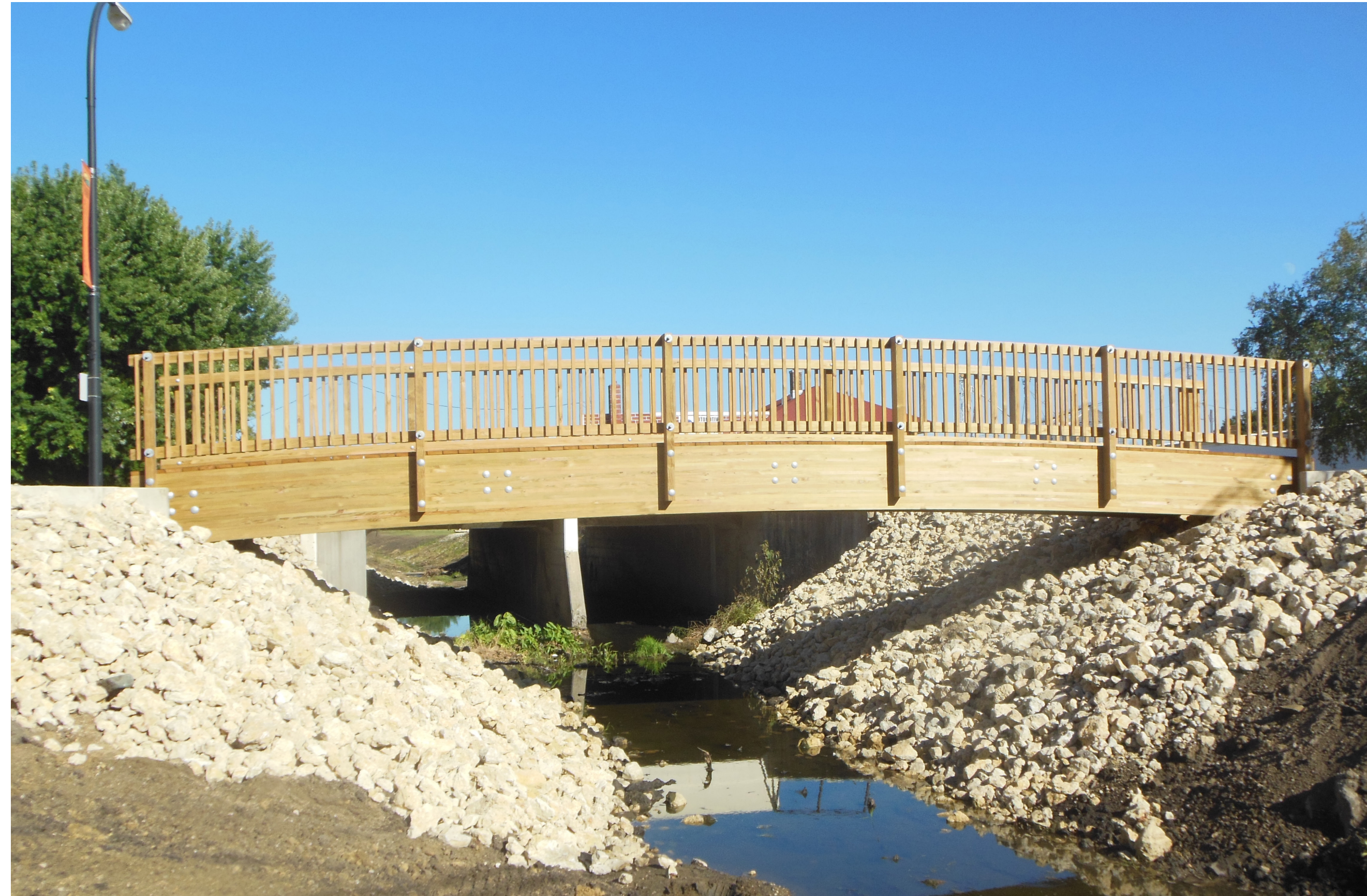
Pedestrian bridge over Sweet Water Creek connecting the community to the trailhead and welcome center
