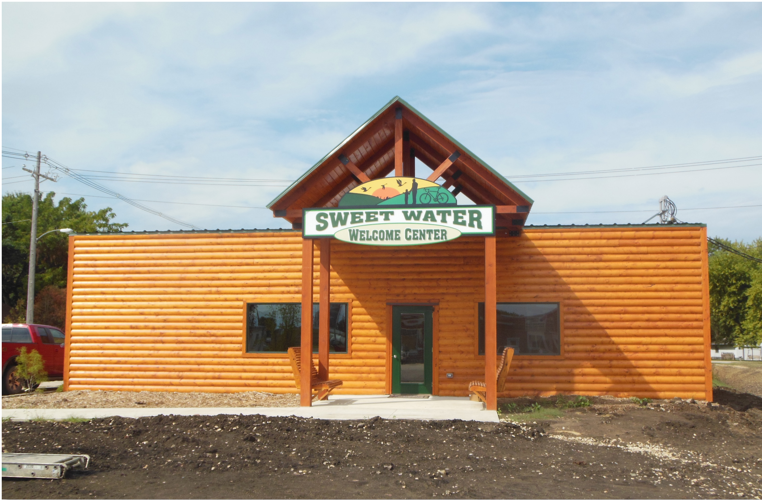
Trailhead welcome center shortly after construction in 2013
