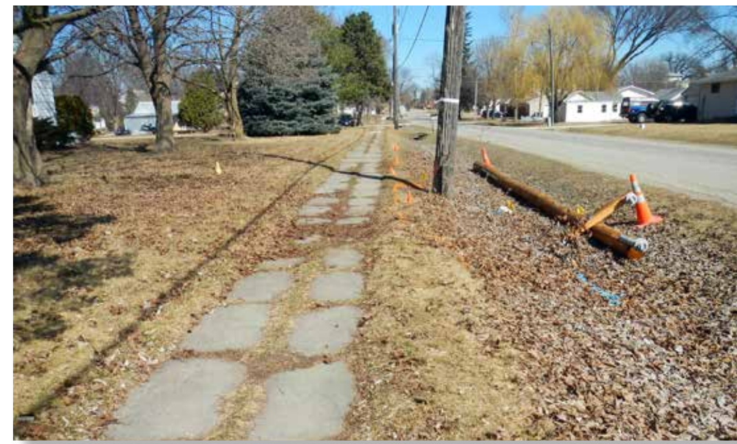
Overgrown and broken sidewalks compromise neighborhood walkability
