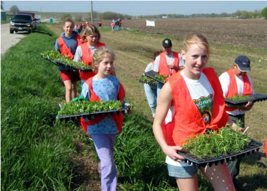
Volunteers plant native vegetation along U.S. Highway 71 near Exira
